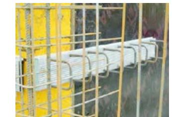
Comfitt - the embedded parts, which accelerate the process of monolithic reinforced concrete construction.
